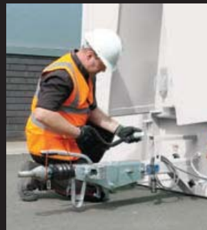
Lower unit to the ground and unplug controls
